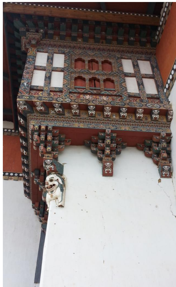
Norbu Bagum below Rabtsel at Gantey Goenpa
