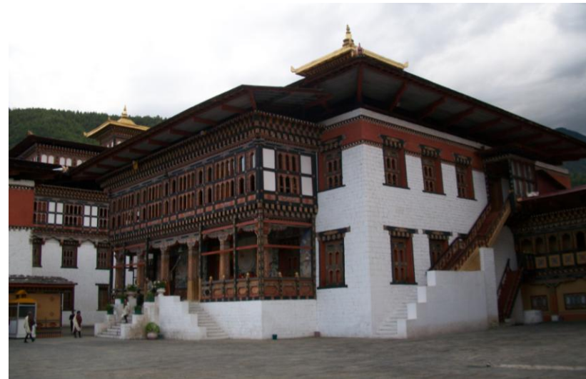
Chenkhep roof over Rabsel at Kunrey of Trashichodtzong in Thimphu (Pictures: Dorji Yangki)
