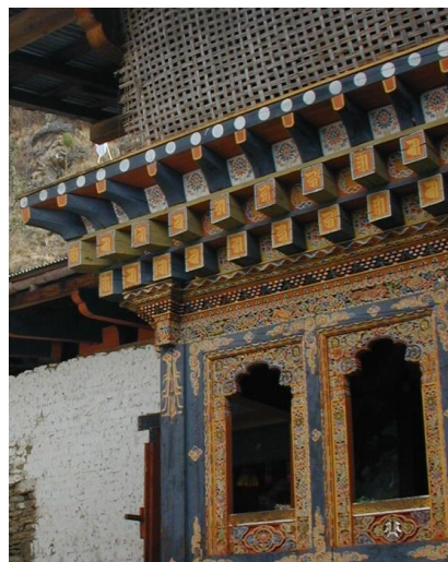
EXAMPLES BOGH AND PHANA IN DIFFERENT BUILDINGS
