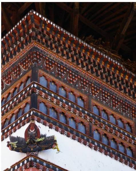
EXAMPLES BOGH AND PHANA IN DIFFERENT BUILDINGS
